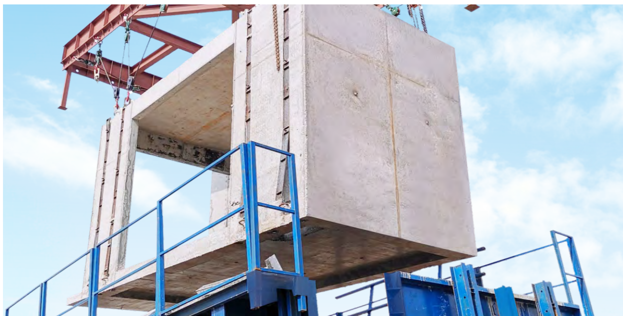
预制房屋 PPVC prefabricated prefinished volumetric construction
